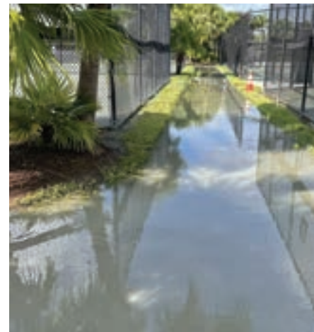
▲ Flooded walkway due to poor drainage
