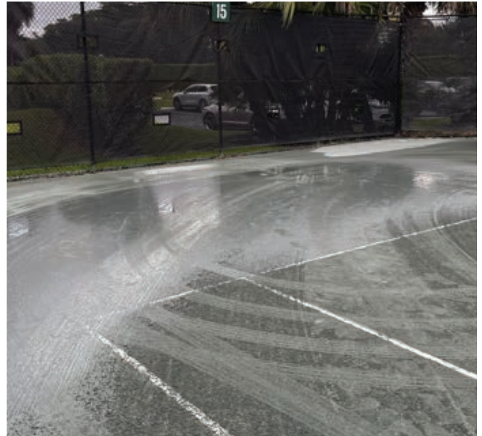
▲ Faulty watering system. Court is both wet and dry at same time
