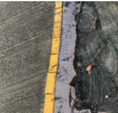
▲ Damaged concrete
