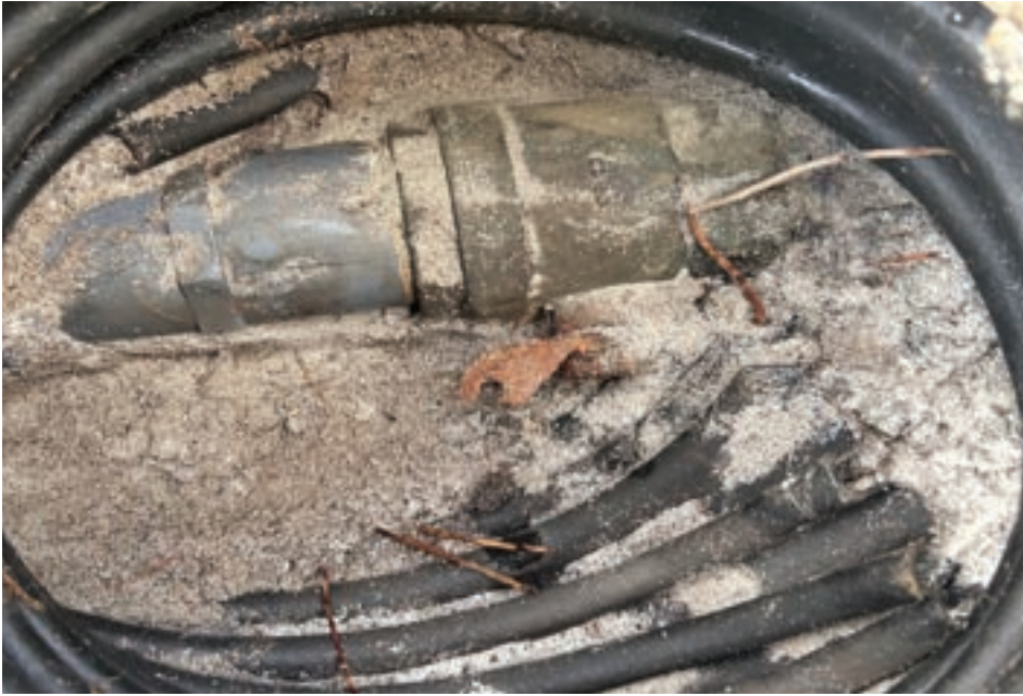
▲ Lateral water line valves are rusted/corroded. Boxes surrounding them are collapsing.
